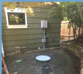
Sewer Cleanout Used for maintenance access to a sewer lateral
