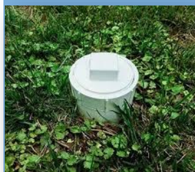
Sewer Cleanout Used for maintenance access to a sewer lateral
